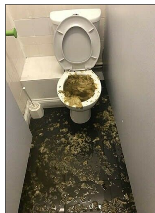
Image: Overflow in a customers home following a sewer line choke
