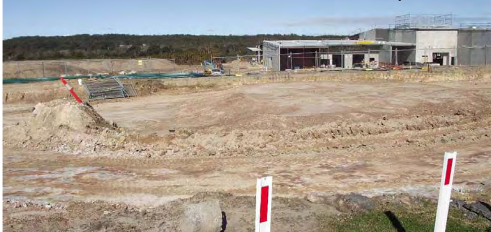
Start of roundabout at Moona Creek Road and Halloran Street Bayswood.
